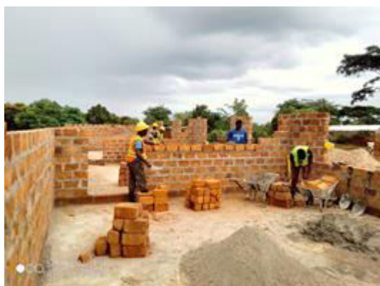
Walls in progress
