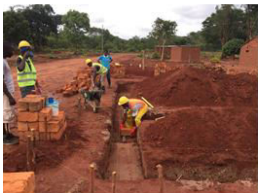
The first brick being laid in the footing
